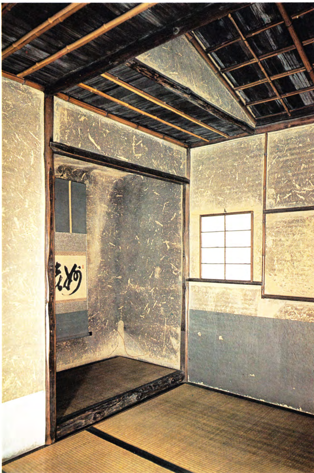
The interior of Taian showing the murodoko alcove with the corner posts plastered over and the ceiling structure.
