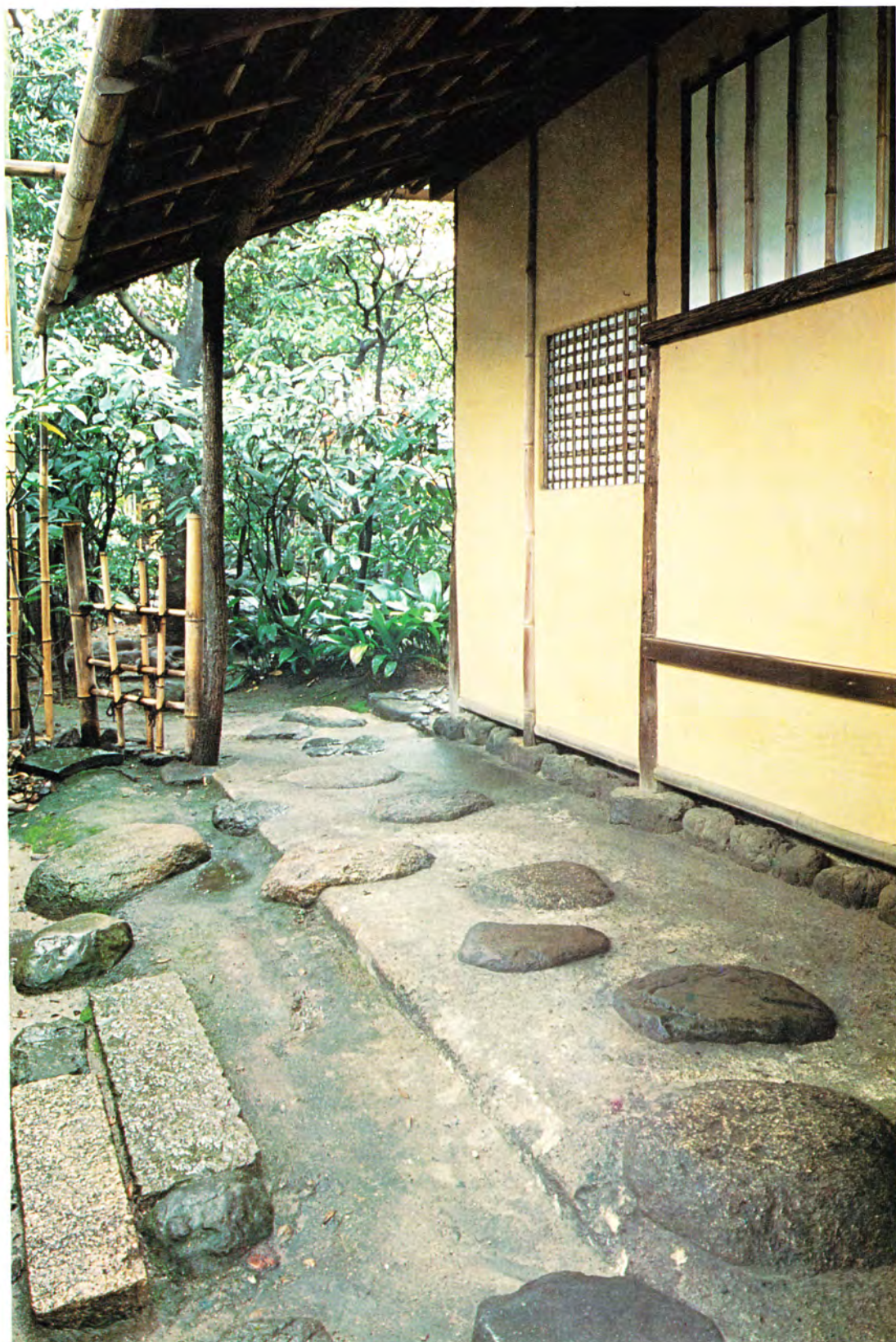
The south side of Taian showing the chikara take , sbitaji mado , renji mado , and path leading to the nijiriguchi .
