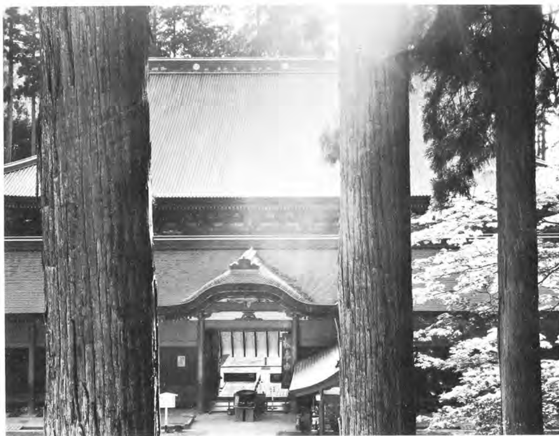
The entrance to the Komponchudō at Enryakuji temple on Mt. Hiei.
