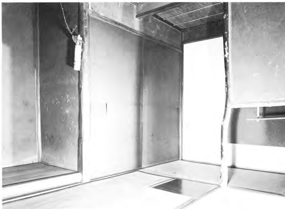
The northeast corner of Shokoken showing the host's entrance in white and the distinctive black-papered panels of the serving entrance.
