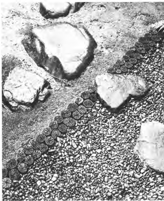
The charcoal that is set into the ground directly beneath the edge of the roof of the Amigasamon at Mushakojisense.
