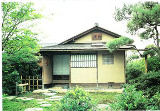
The south exterior wall of Jo-an showing the distinctive earthen area in front of the entrance and the circular openwork window in the sleeve wall on the right. (Uraku-en, Inuyama)
