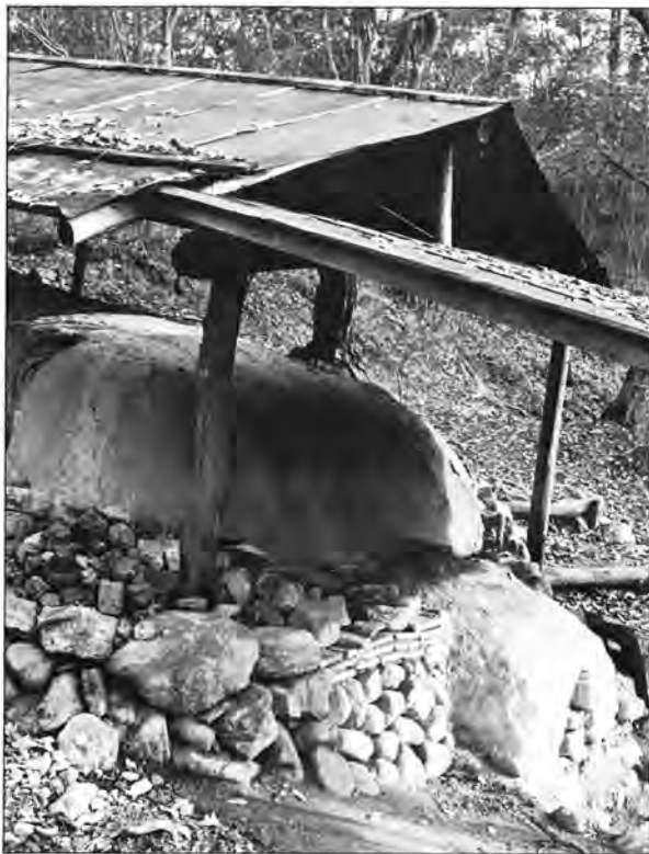
Working replica of a Momoyama-period Shino kiln, constructed by Arakawa Toyozo in 1933. Photo courtesy of Kusunishi Sosei, Nara.
