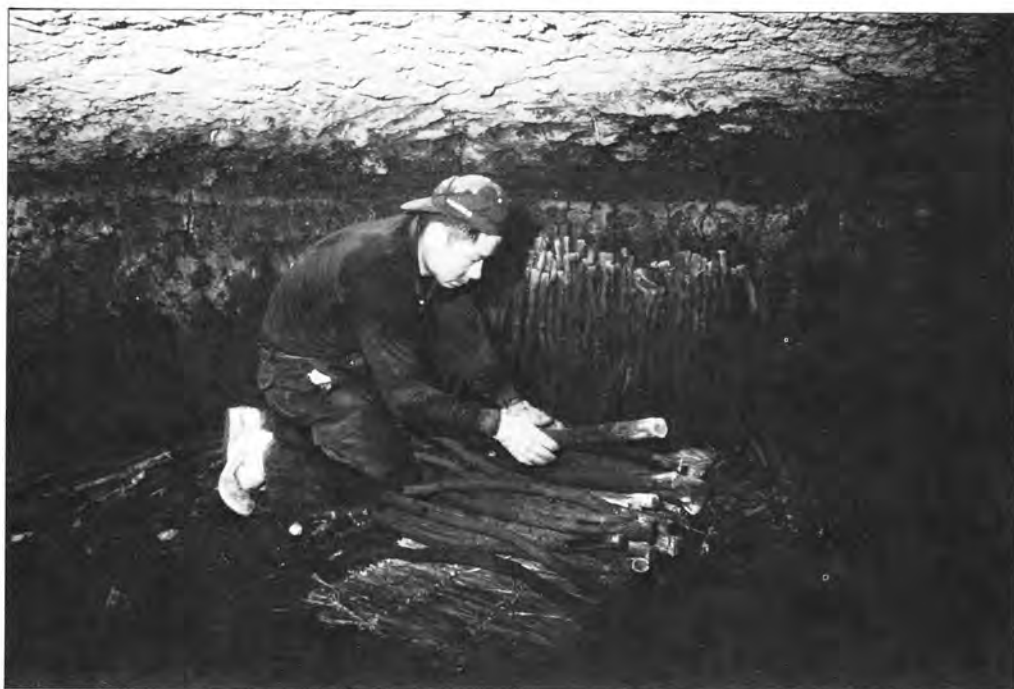
Above: Removing the sumi from the kiln. The interior of the kiln is still extremely hot. Within this, the sumi-maker carefully places each piece, one by one, on a straw mat, and bundles them. An average batch yields about fifty bundles. Below: The bundled sumi, ready to be taken to market. The best pieces have a fine "chrysanthemum" pattern at the cross-section, with bark firmly intact.
