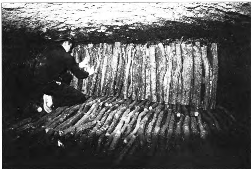
Above: Overall view of a typical kuro-zumi kiln site, with firewood piled high. In the past, almost all sumi kilns were located deep in the mountains. Nowadays, many are located on flatland. Below: Placing the wood in the kiln. Because the pieces placed in the front tend to carbonize irregularly, the best pieces—those to be used for chanoyu—are placed toward the back of the kiln.
