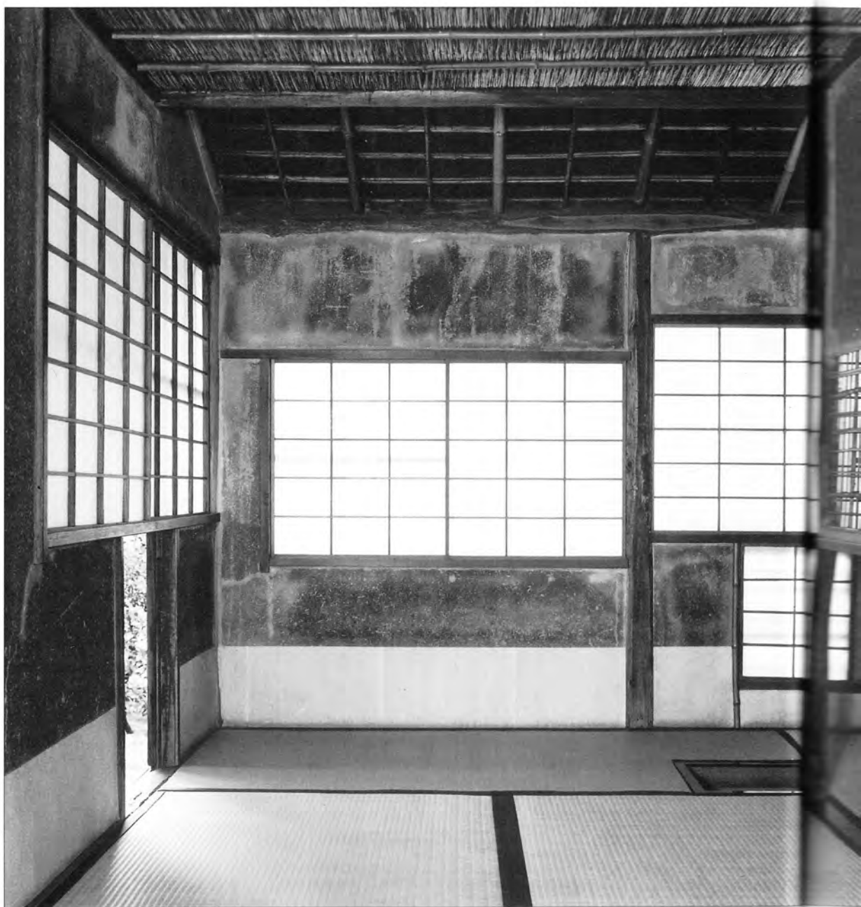
Tearoom known as the Konchi'in Hasso-no-seki; north wall. At the Konchi'in subtemple of Nanzenji temple, Kyoto. Built ca. 1628; design by Kobori Enshu. Though called an "eight-windowed" room, there are actually only six windows, all visible in the above photograph. Important Cultural Property.
