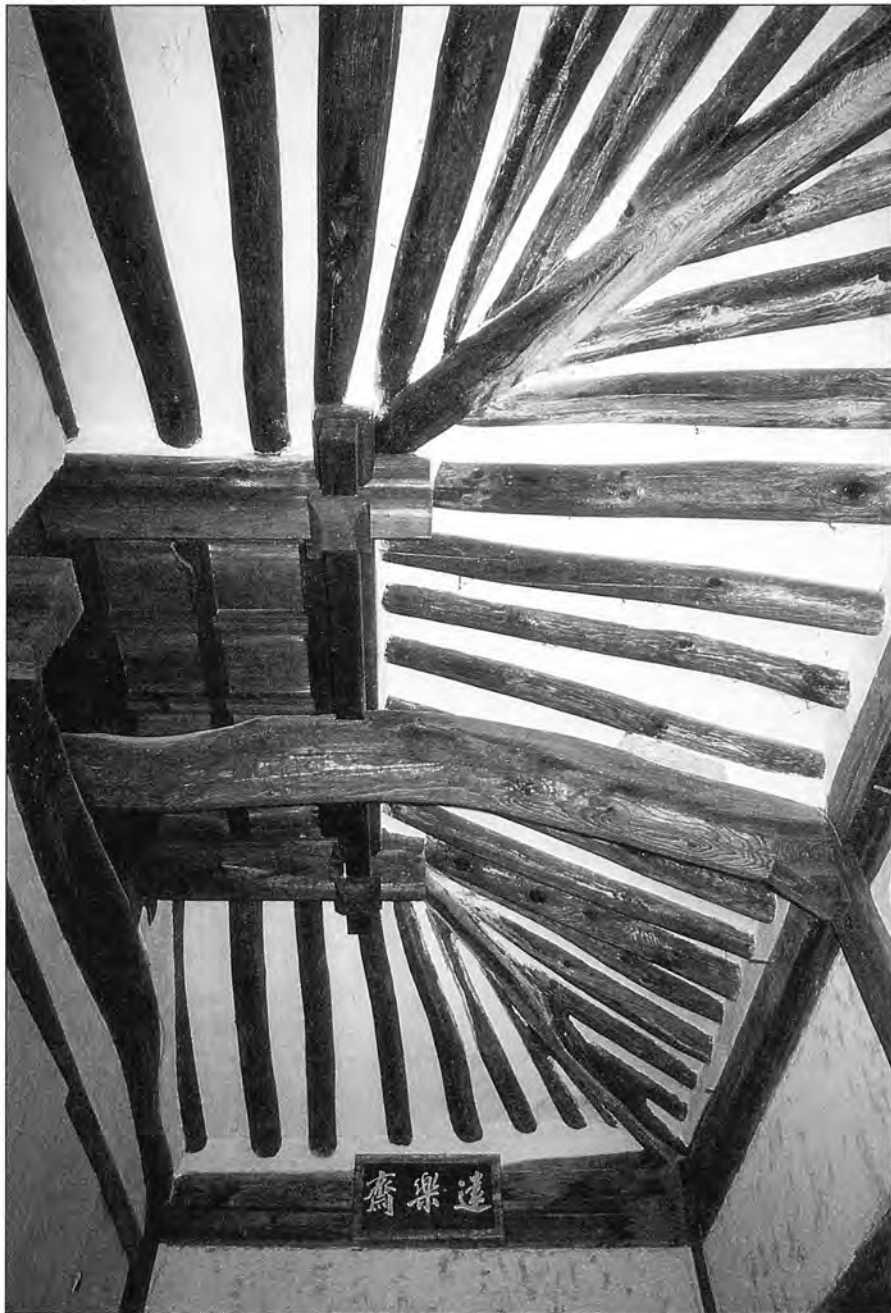
Ceiling in the former country house of a Korean aristocrat. Typical of traditional Korean residential architecture, there are no ceiling boards and the wooden roof beams are visible. In Japan, this kind of ceiling, termed funazoko-gata (ship's-bottom style), is sometimes seen in rustic tearooms.
