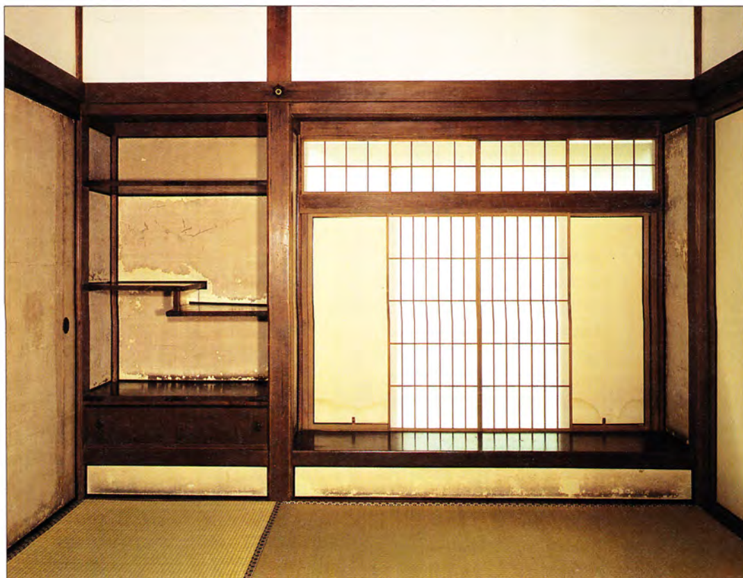
The Dōjinsai room within the Tōgudō hall at Jishōji temple. It has built-in staggered shelves ( chigaidana ) and, in front of the window, a built-in shoin desk —the fixture that is the namesake of shoin rooms and shoin architecture.
